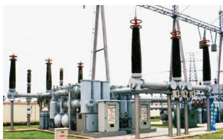
ZF11-252 气体绝缘金属封闭开关设备 (GIS) ZF11-252 gas-insulated metal-enclosed switchgear (GIS)
