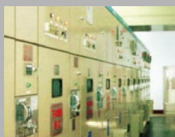
XGN2-12型 箱型固定式金属封闭开关柜 XGN2-12 box fixed metal-enclosed switch cabinet
