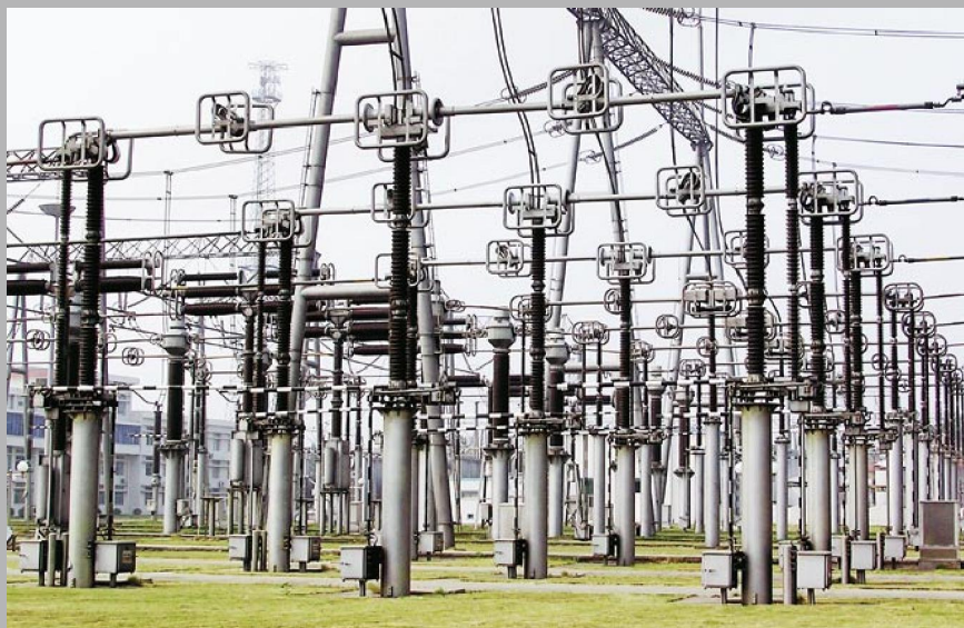
GW28/29型系列高压隔离开关 额定电压：252kV/363kV/550kV GW28/29 series of disconnectors Rated voltage: 252kV/363kV/550kV
