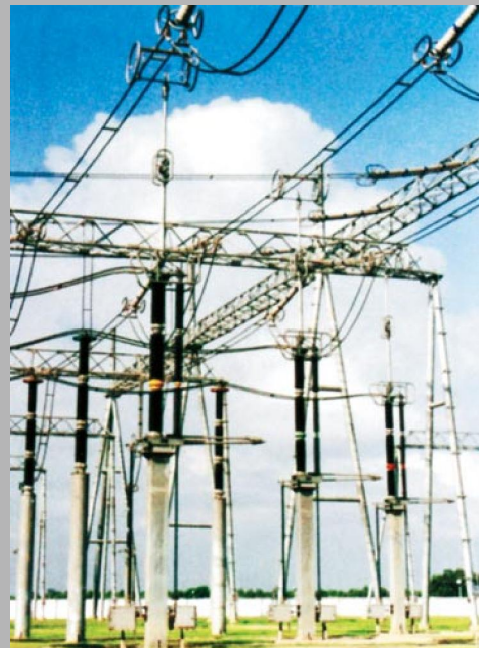
GW16B/17B型系列高压隔离开关 额定电压：126kV/252kV/363kV/550kV GW16/17B series of disconnectors Rated voltage: 126kV/252kV/363kV/550kV
