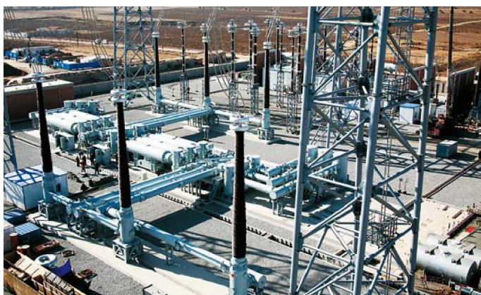
ZF27-1100 气体绝缘金属封闭开关设备 (GIS) ZF27-1100 gas-insulated metal-enclosed switchgear (GIS)
