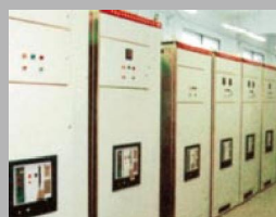
MNS型低压抽出式开关柜 MNS low voltage draw-out switch cabinet
