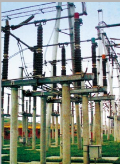
GW7型系列高压隔离开关 额定电压：40.5kV/72.5kV/126kV/ 145kV/252kV GW7 series of disconnectors Rated voltage: 40.5kV/72.5kV/126kV/145kV/252kV
