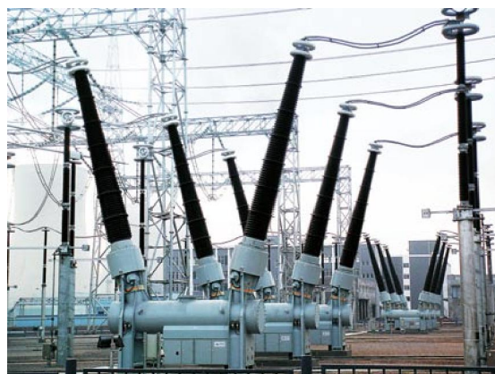
LW55-800 罐式断路器 LW55-800 dead tank circuit breaker
