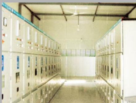
KYN28A-12型 铠装移开式金属封闭开关柜 KYN28A-12 metal-clad switch cabinet
