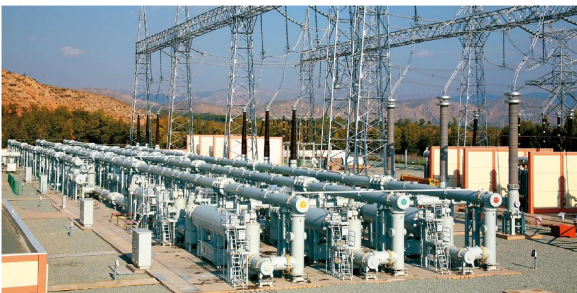
ZF27-800 气体绝缘金属封闭开关设备 (GIS) ZF27-800 gas-insulated metal-enclosed switchgear (GIS)
